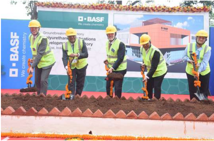
Your Company broke ground on its new Polyurethane Application Development Laboratory in October 2022. To be inaugurated in 2024, the lab will strengthen collaboration with Indian customers from high-growth industries including consumer appliances, construction, footwear, furniture, and transportation.
